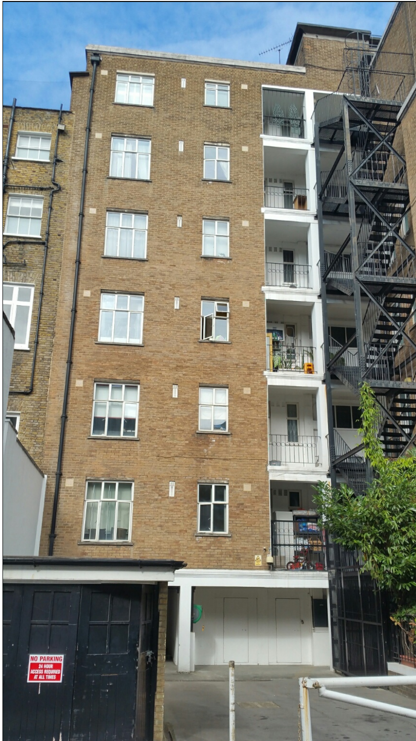
Rear of Montagu Court viewed from Gloucester Place Mews
